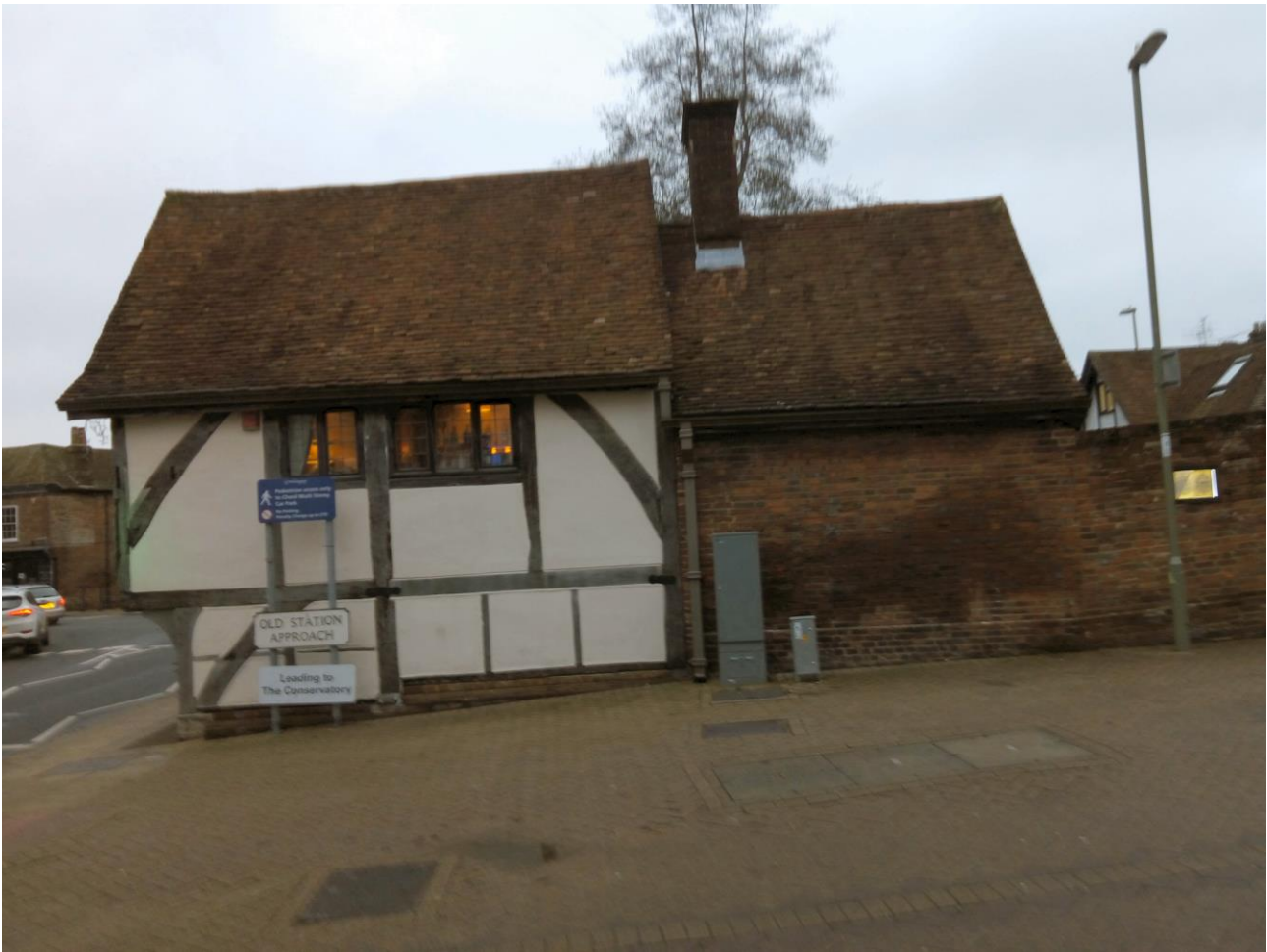
View of 1 Chesil Street from South 1
