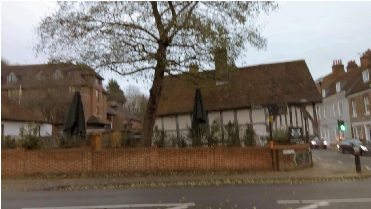
View of 1 Chesil Street from South 3
