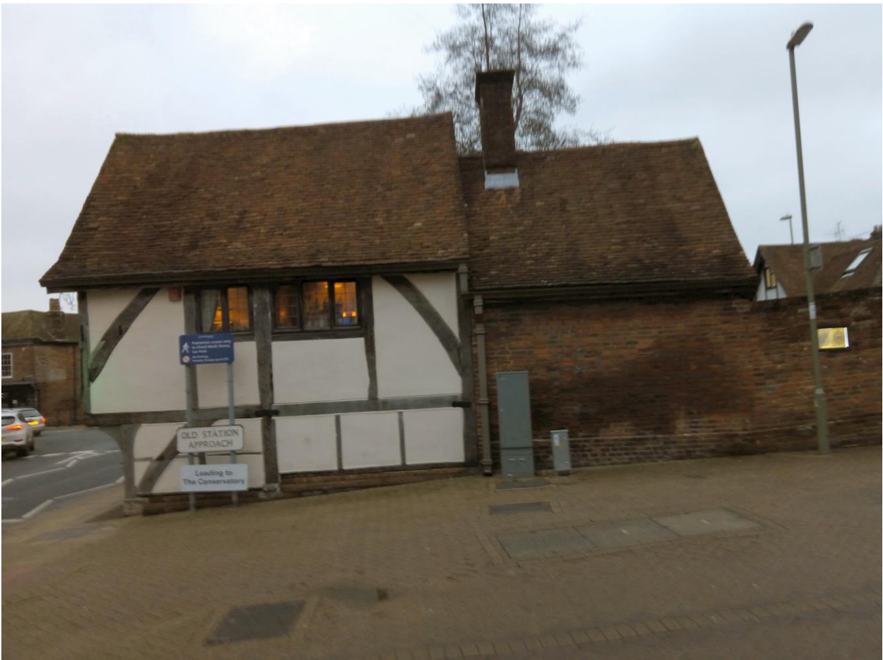
View of 1 Chesil Street from South 2
