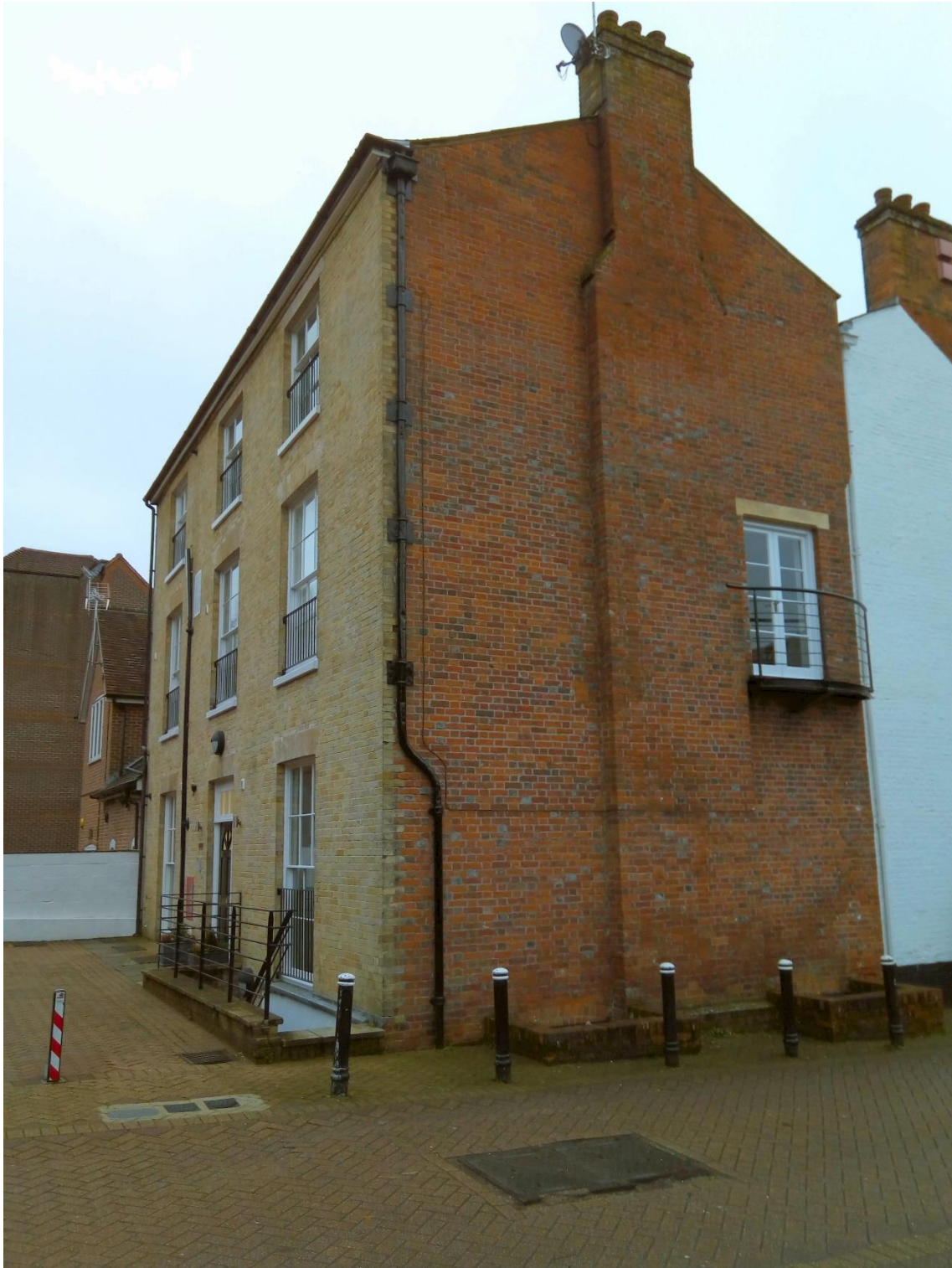
View of 3 Chesil Street from North East
