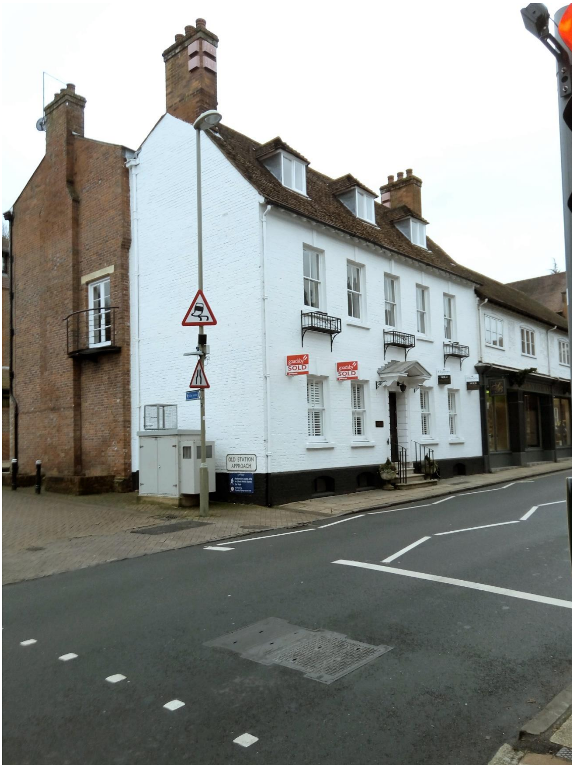
View of 3 Chesil Street from North West
