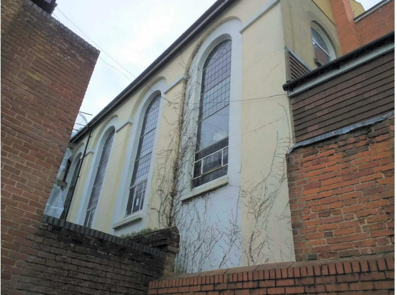
Winchester Baptist Church viewed from Swan Lane 1
