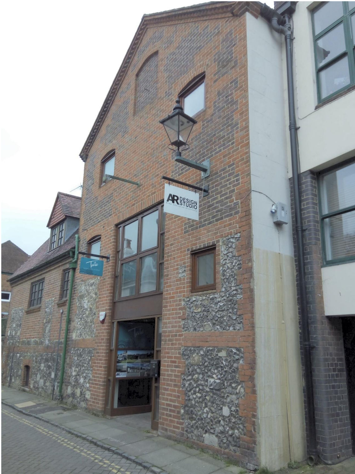
Calpe House rear view from Little Minster Street 4
