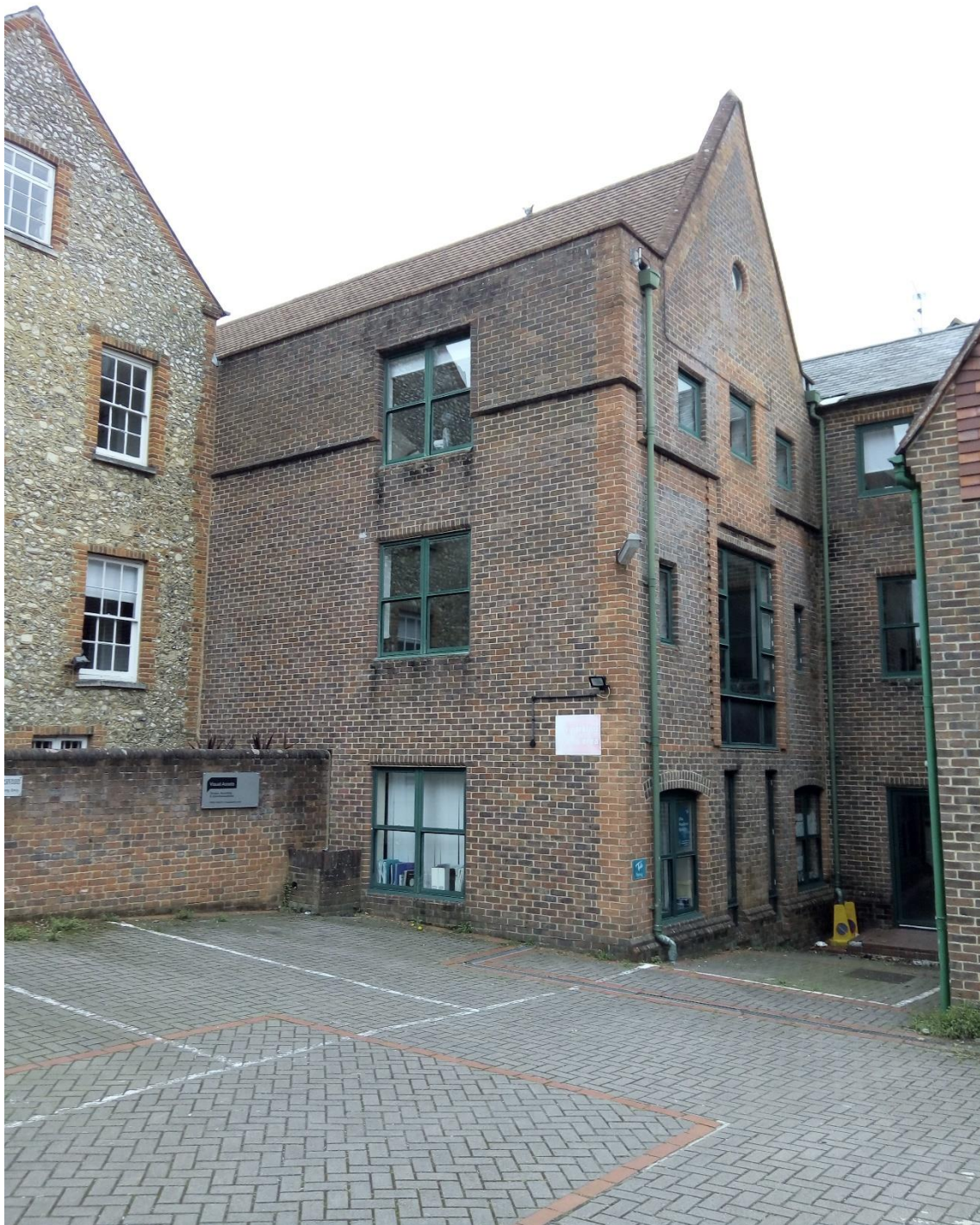
Calpe House rear view from Little Minster Street 2
