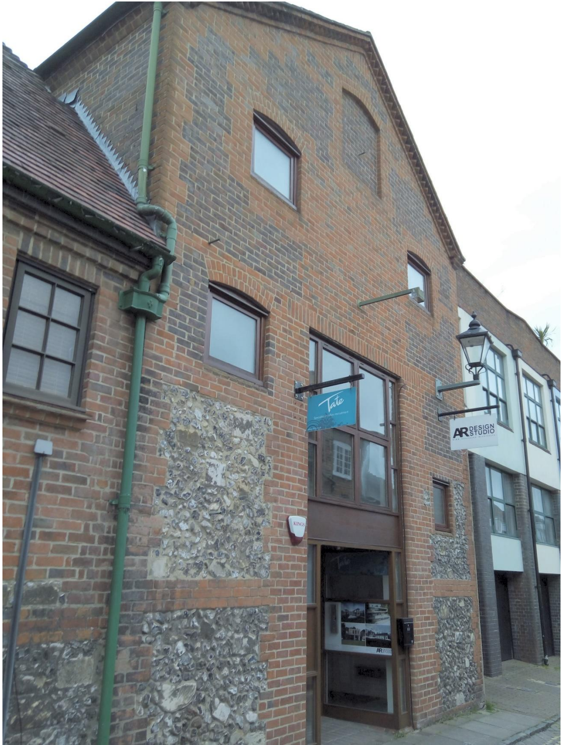
Calpe House rear view from Little Minster Street 3
