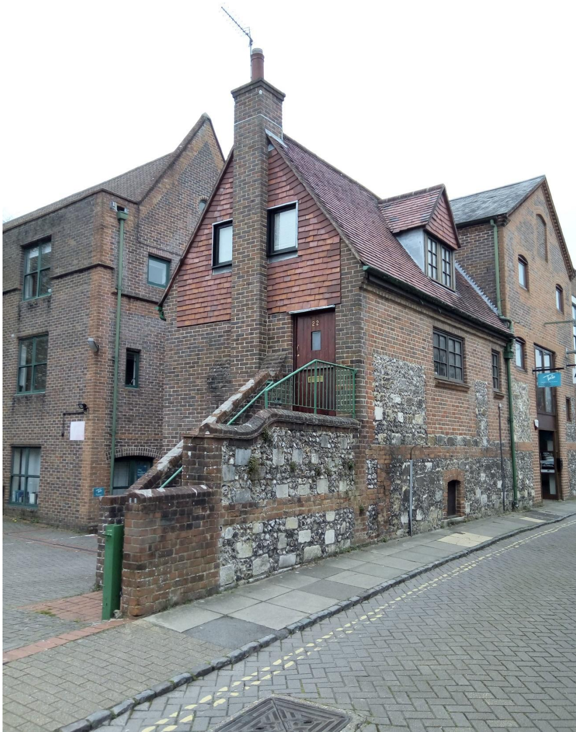
Calpe House rear view from Little Minster Street 5
