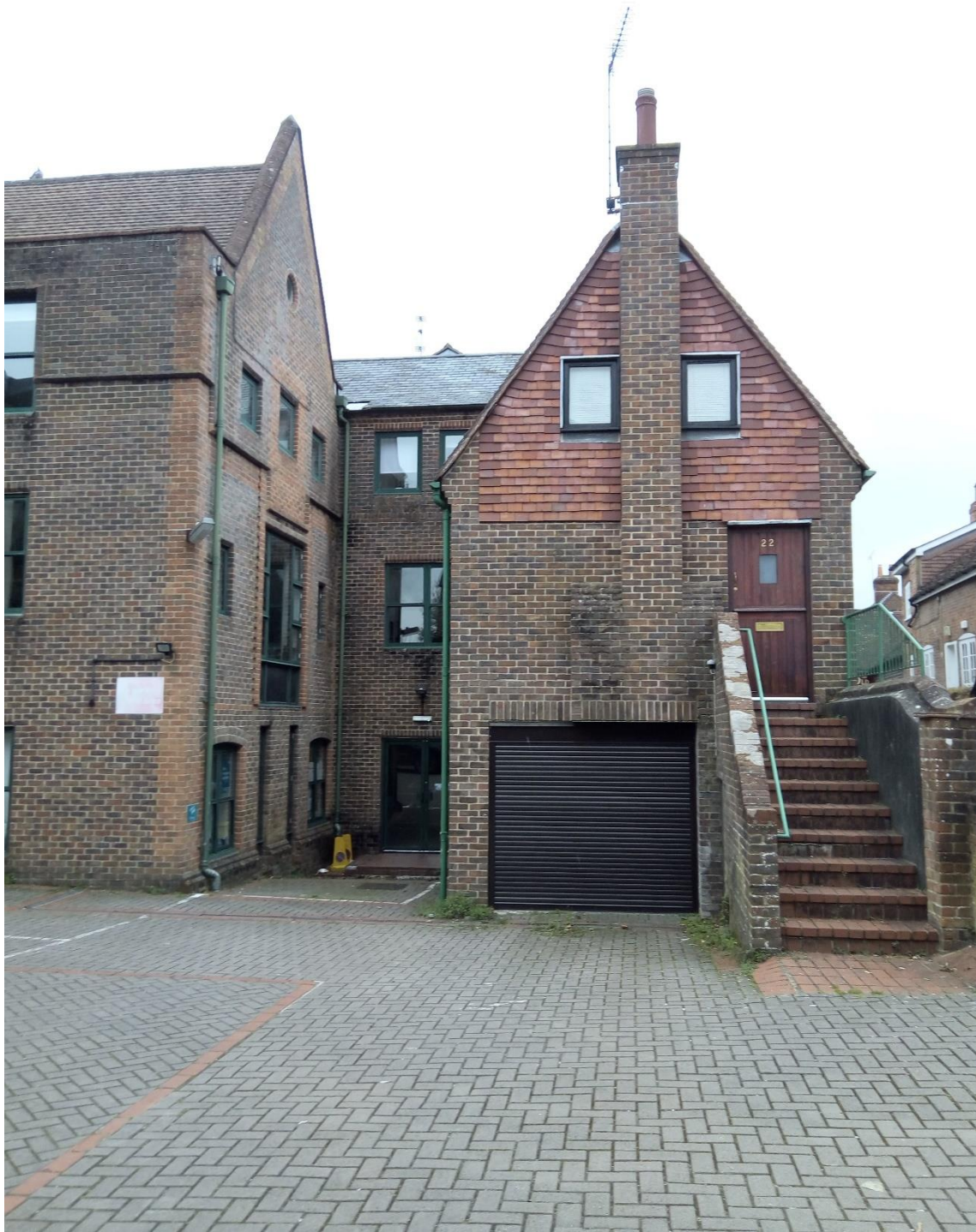
Calpe House rear view from Little Minster Street 1
