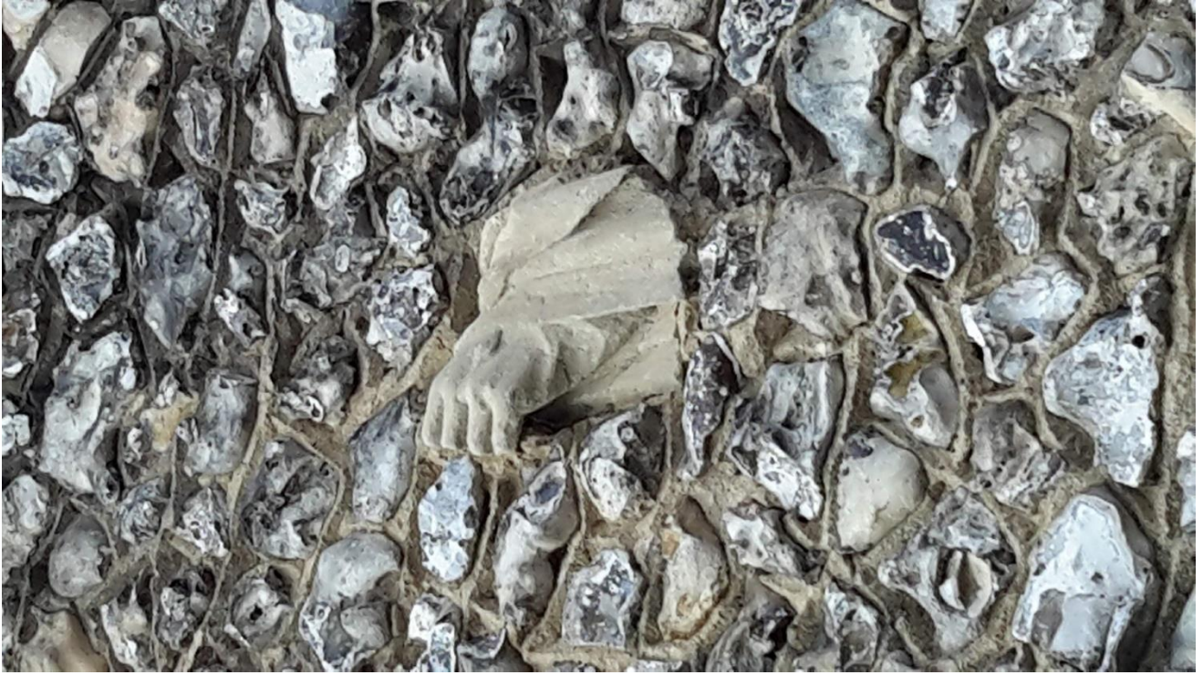
Holy Trinity Church Wall Showing Reused Stone 2
