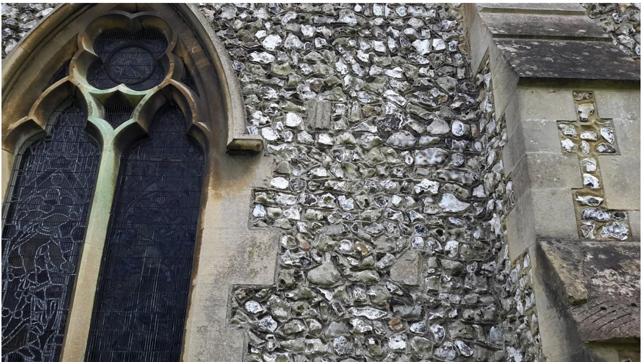
Holy Trinity Church Wall Showing Reused Stone 1
