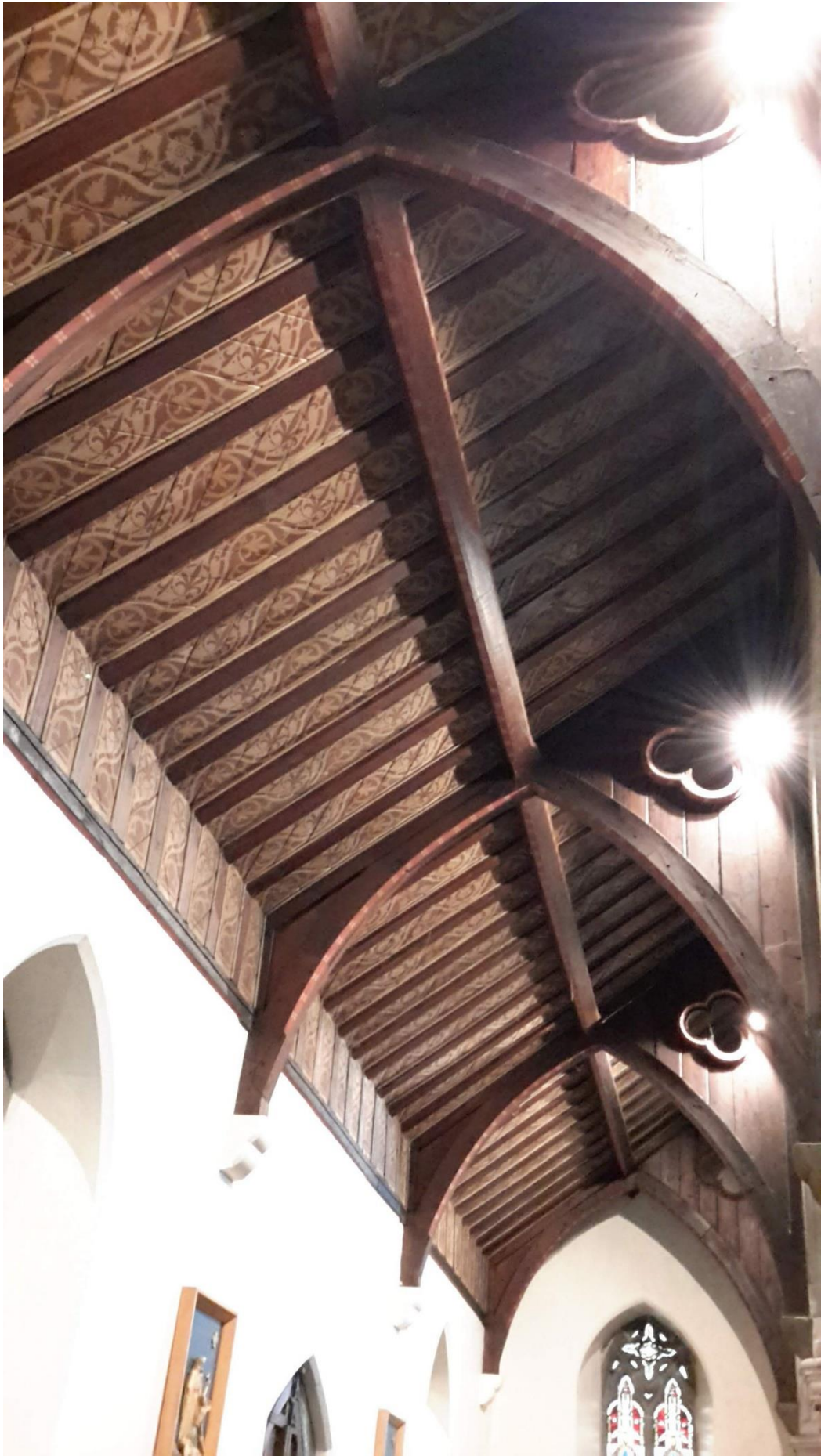
Holy Trinity Church Roof Detail
