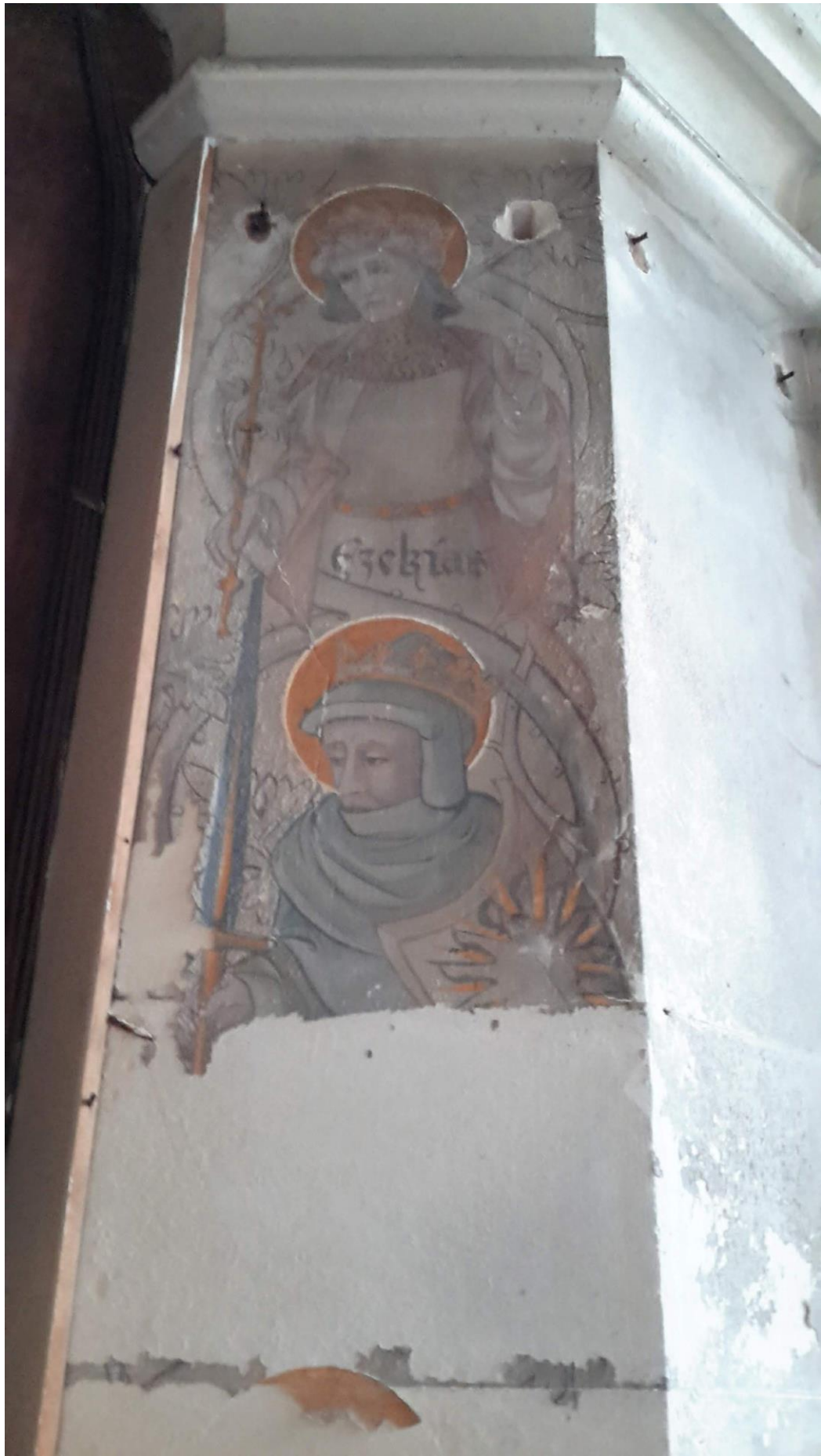
Holy Trinity Church Remains of Painted Wall
