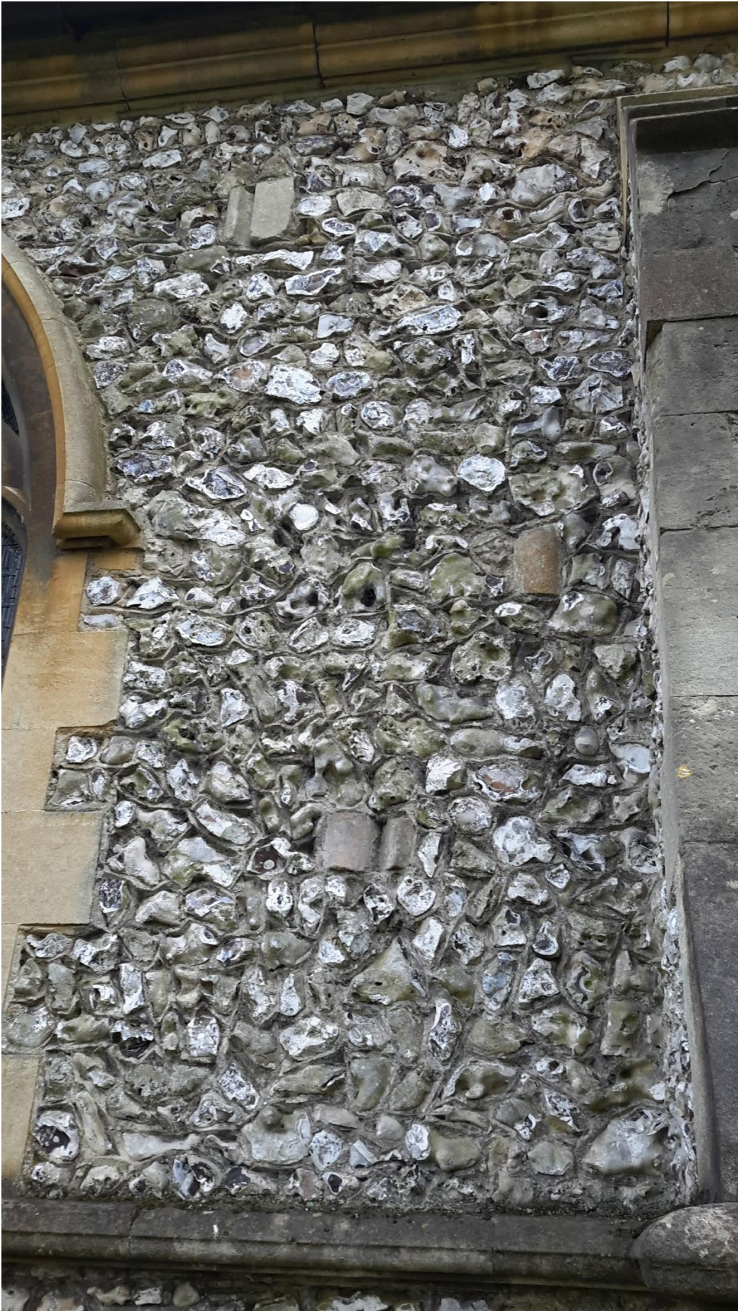
Holy Trinity Church Wall Showing Reused Stone 3
