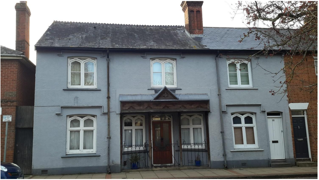
Holy Trinity Church House Belonging to Church
