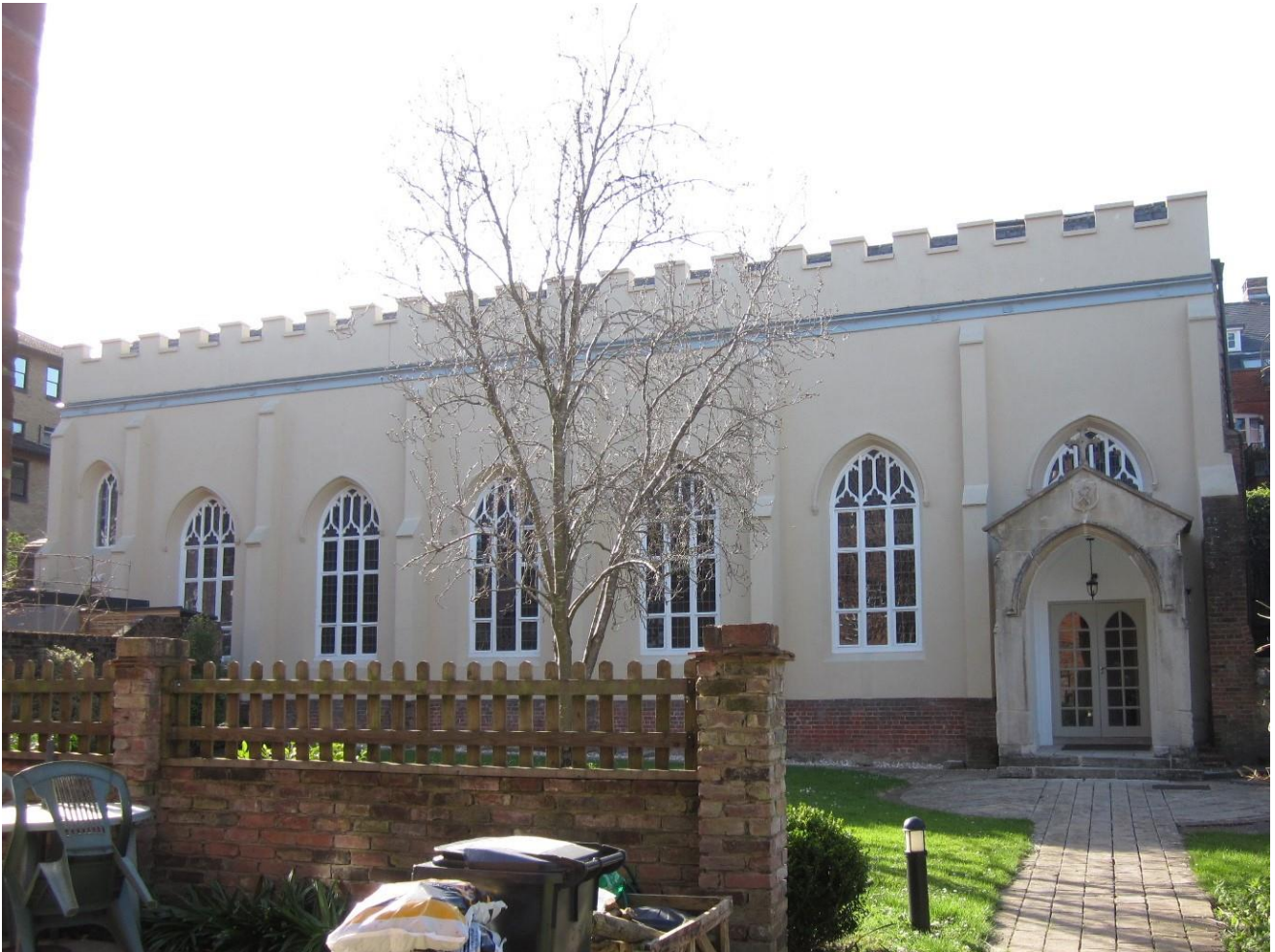
Milner Hall North Side
