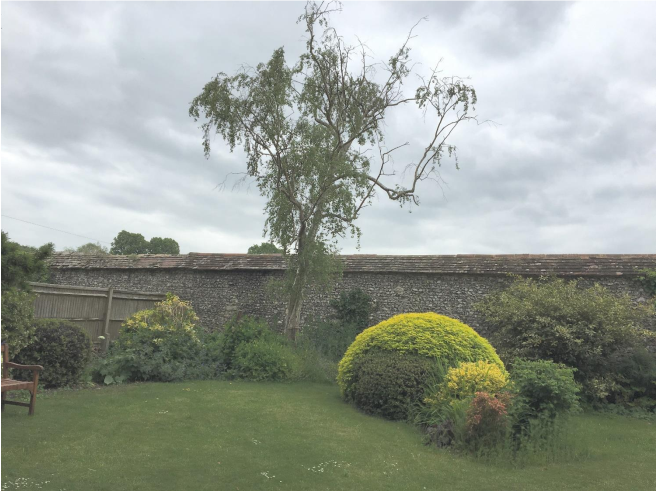
Quaker Meeting House wall at rear of garden
