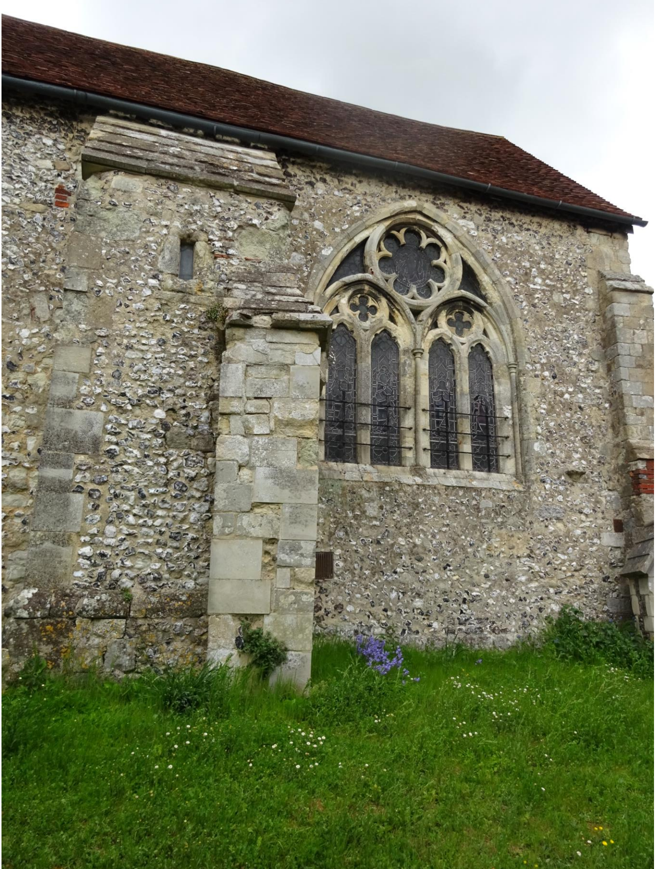
Church of St John The Baptist, exterior window
