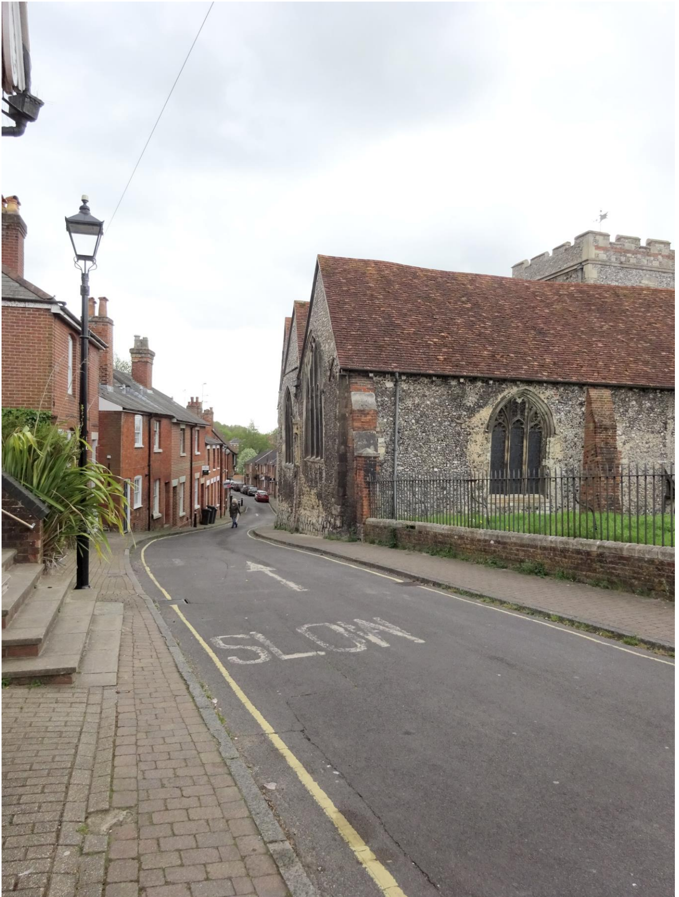
Church of St John The Baptist, view from North of St John's Street 2
