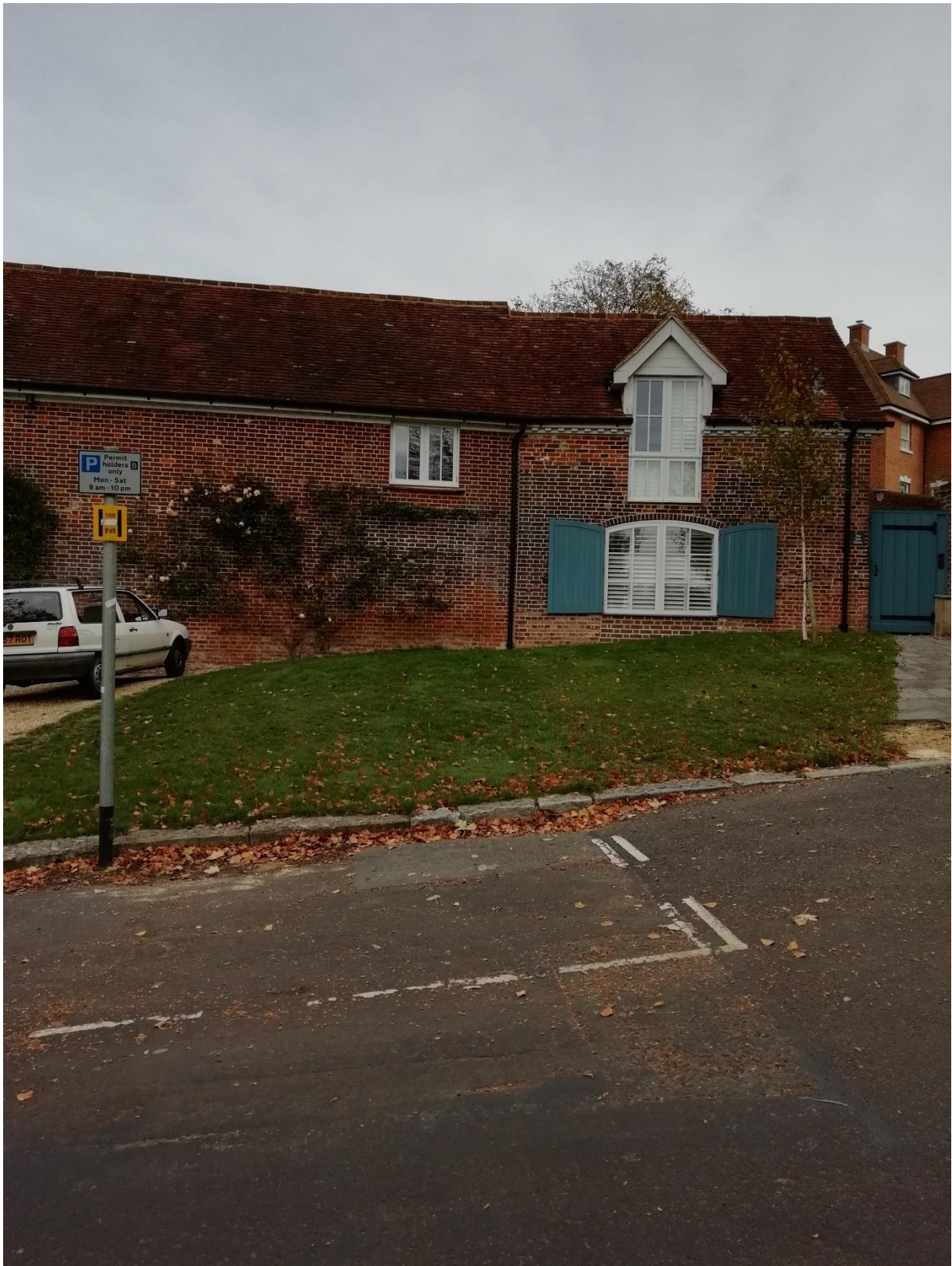
Stable Block, St John's Croft
