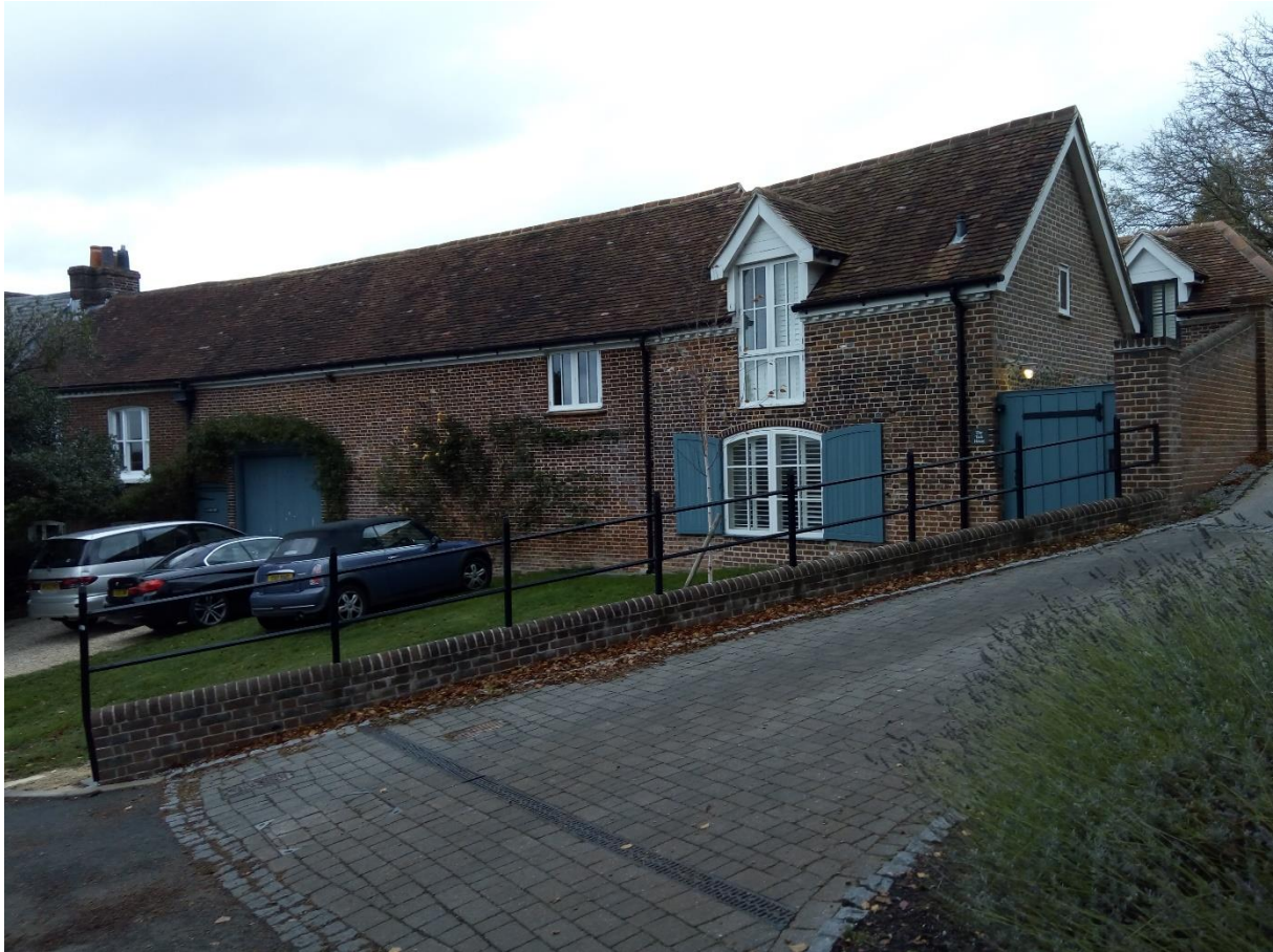
Stable Block, St John's Croft
