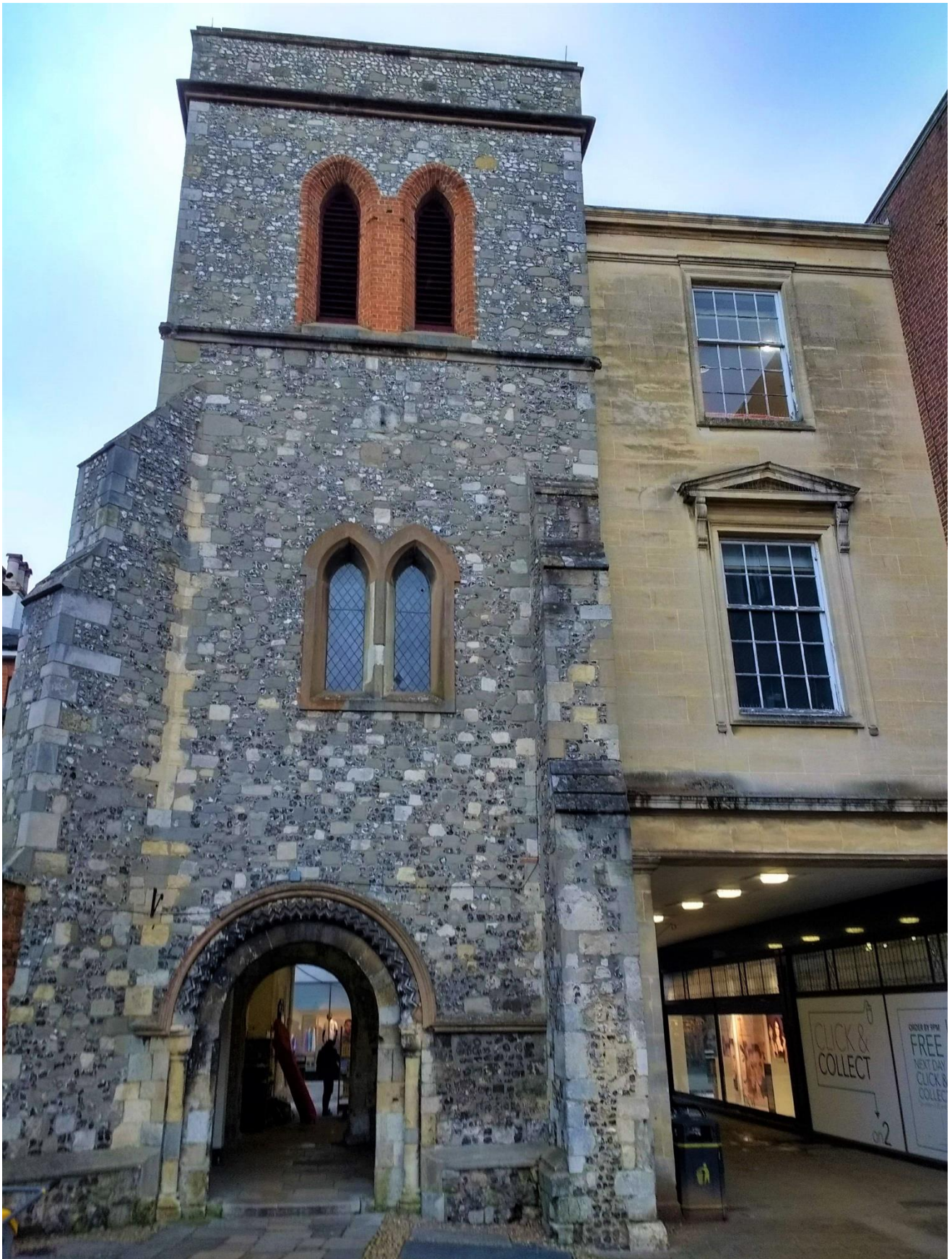
St Maurice Tower from Cathedral Side
