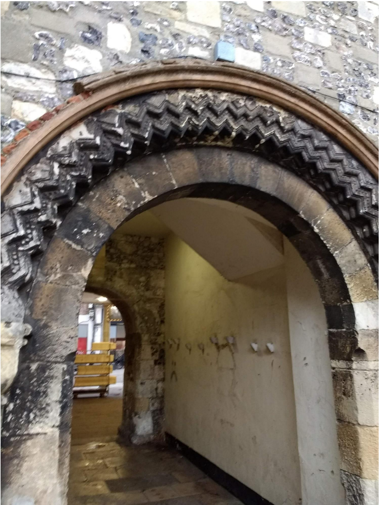
St Maurice Covert right hand arch from Cathedral Side
