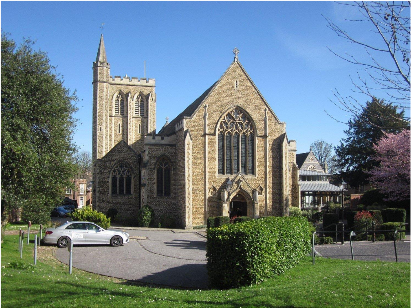
St Peter's Church North West View
