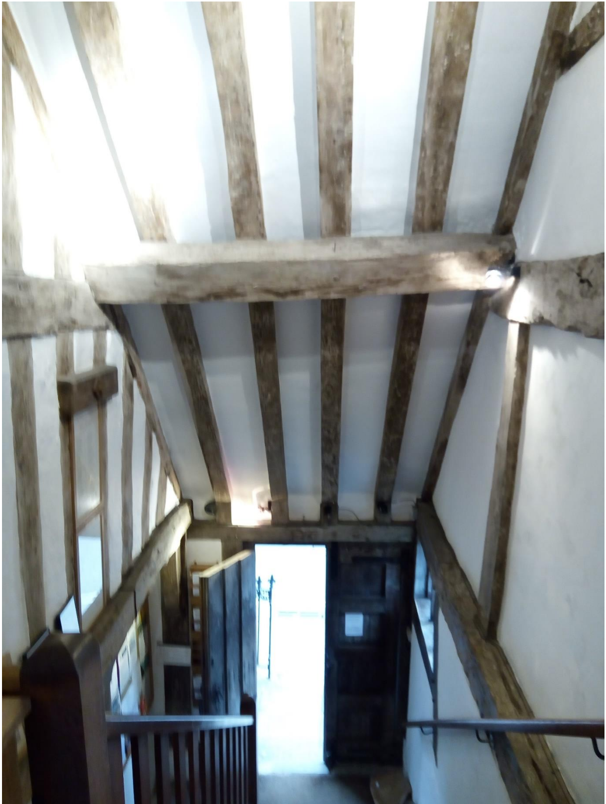
St Swithun Church Interior – Ceiling
