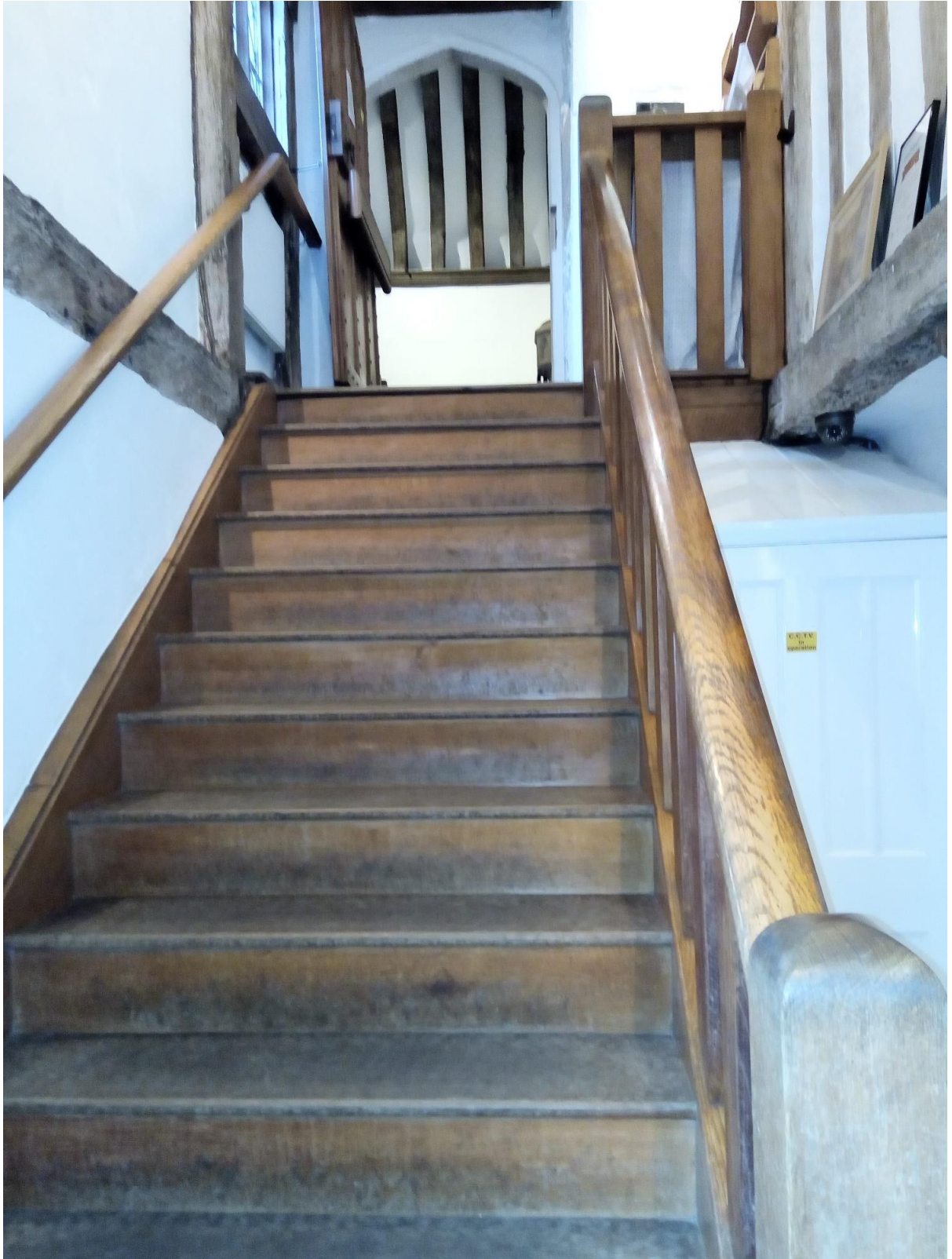
St Swithun Church Interior – Staircase
