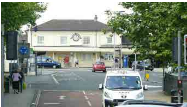
Winchester Station Building: View of Station frontage and forecourt
