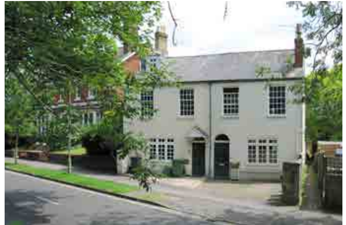
Worthy Lane: Terrace forms part of the Hyde Conservation Area
