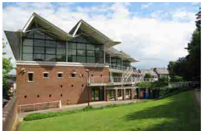
Hampshire Records Office: Well liked local modern building
