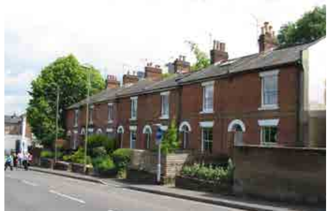
Gladstone Street: Simple terrace in good condition
