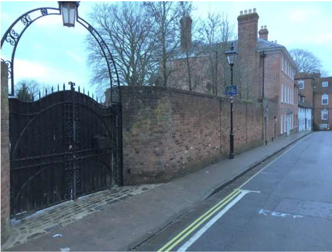
Wall of 13 St Thomas Street 2
