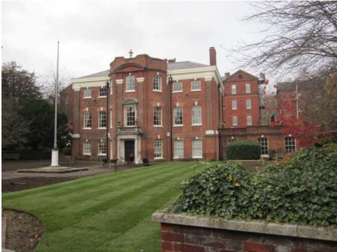
Serle's House, Southgate Street
