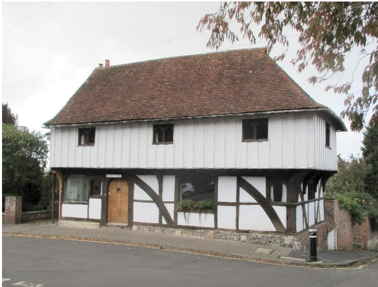
24-25 St Johns Street from East
