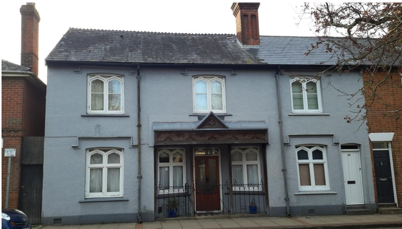
119 – 121 Upper Brook Street
