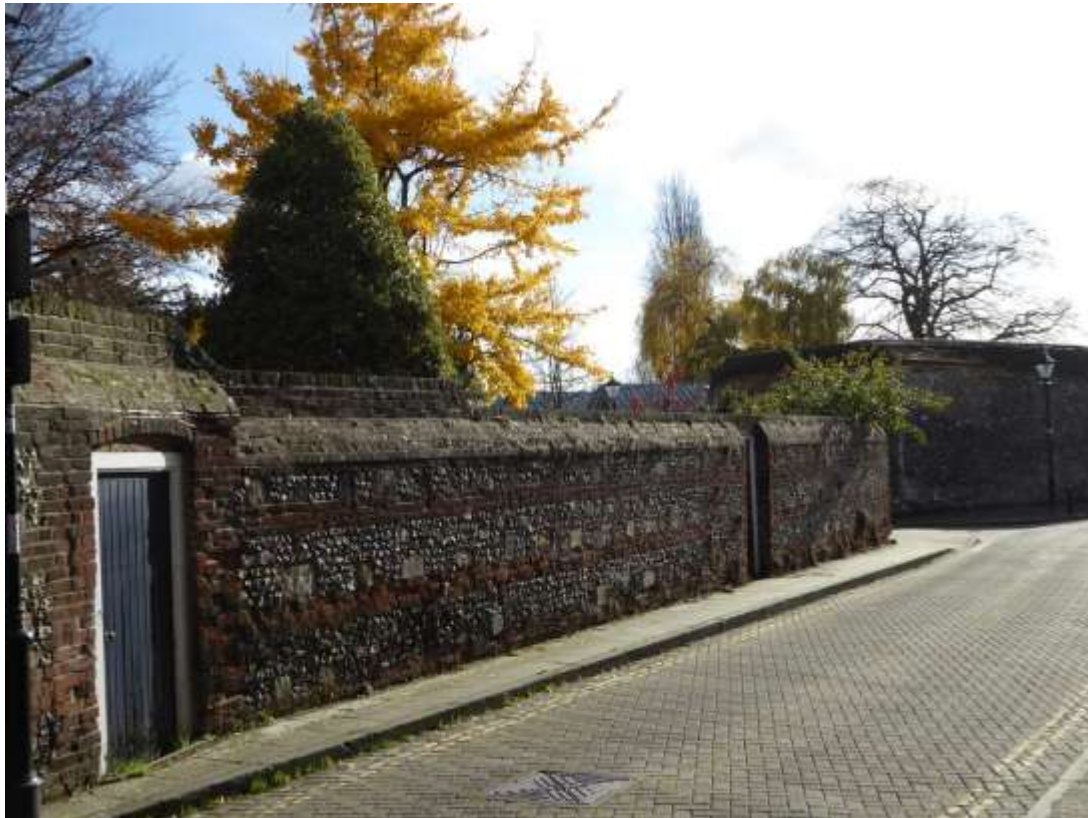
Garden wall of Minster House, 3 Great Minster Street
